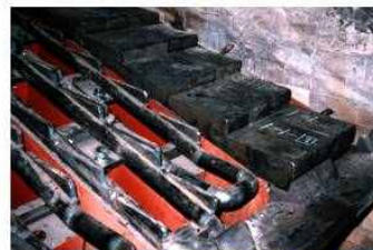
(Water tube under Grate)
